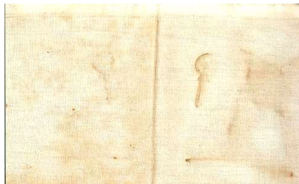
Figure 8 Internal surface (two days before the earthquake of 10-09-2000, Torre Pellice, of magnitudo 3.2 and depth 12 Km), water imbibition
